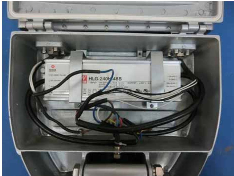
Photo 3 Internal view of EUT
